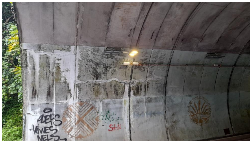
Tunnel de la pointe Arahoro – Fissuration
